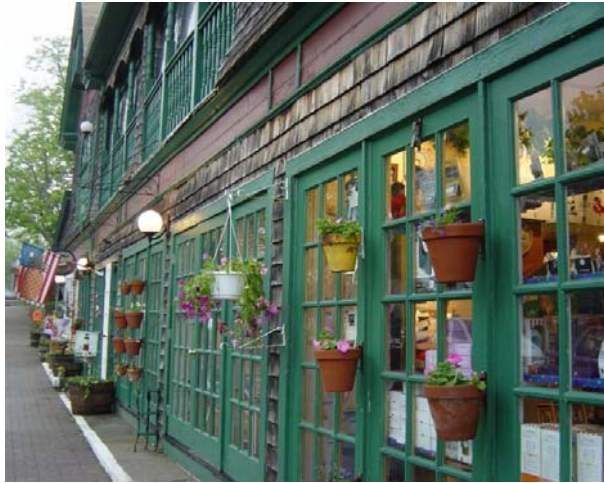
Ground floor multi-pane windows
