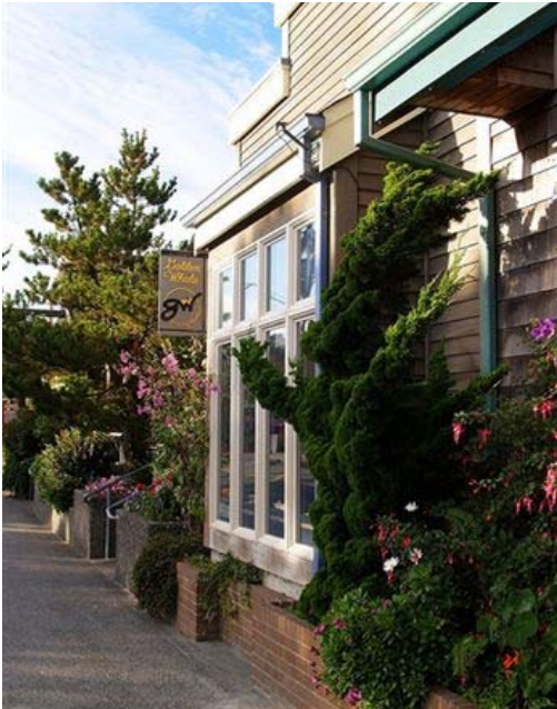
Varied rooflines, materials and window projections make for a successful facade.
