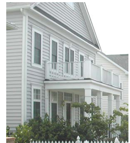
Architectural detailing frames roof, façade, and windows.
